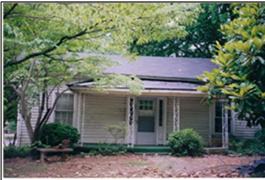
The house in its second location (1910-2005)
